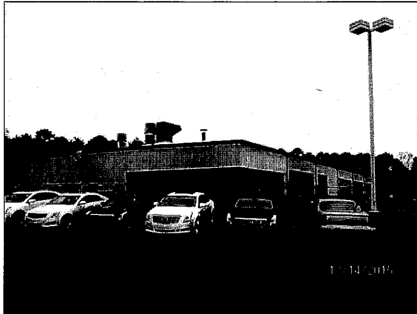
Existing collision center in the southern corner of the property.
